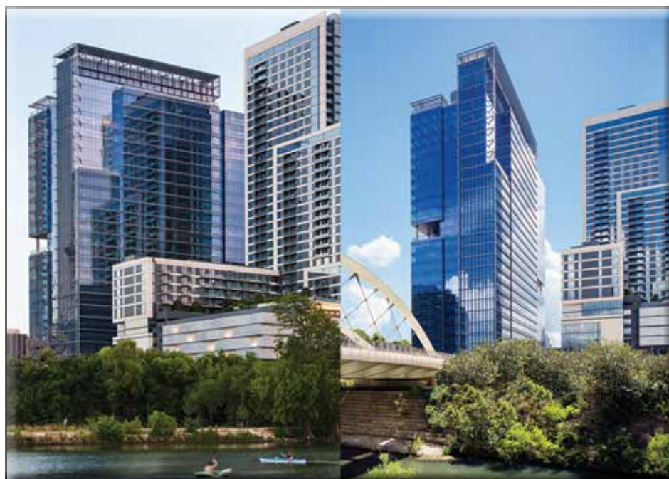
500 West 2nd Street exterior view overlooking Lady Bird Lake
